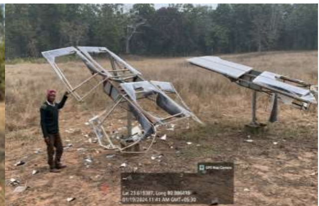
Solar panel damaged by Elephant group in BTR
